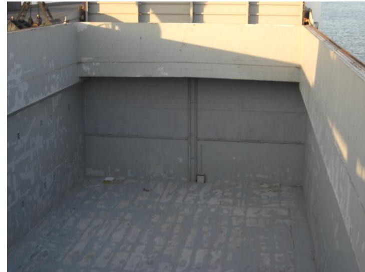
BACKSIDE OF HOLD NO.2
