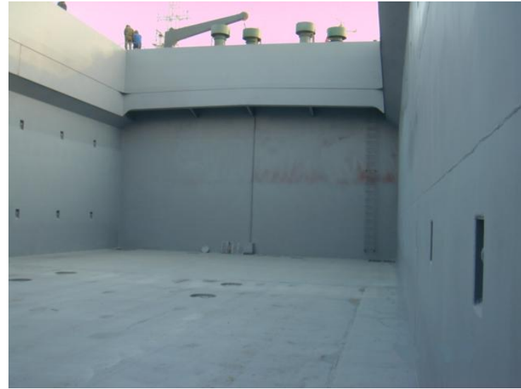
BACKSIDE OF HOLD NO.1
